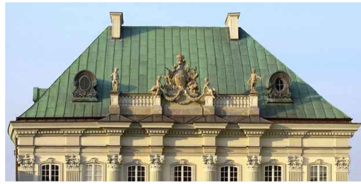
COPPER ROOF REFERENCE
